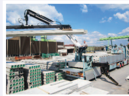
Concrete floor panels handling
