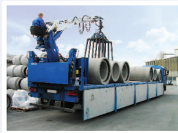
Sewage pipe handling
