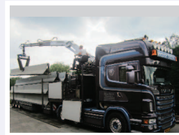
Road barrier handling
